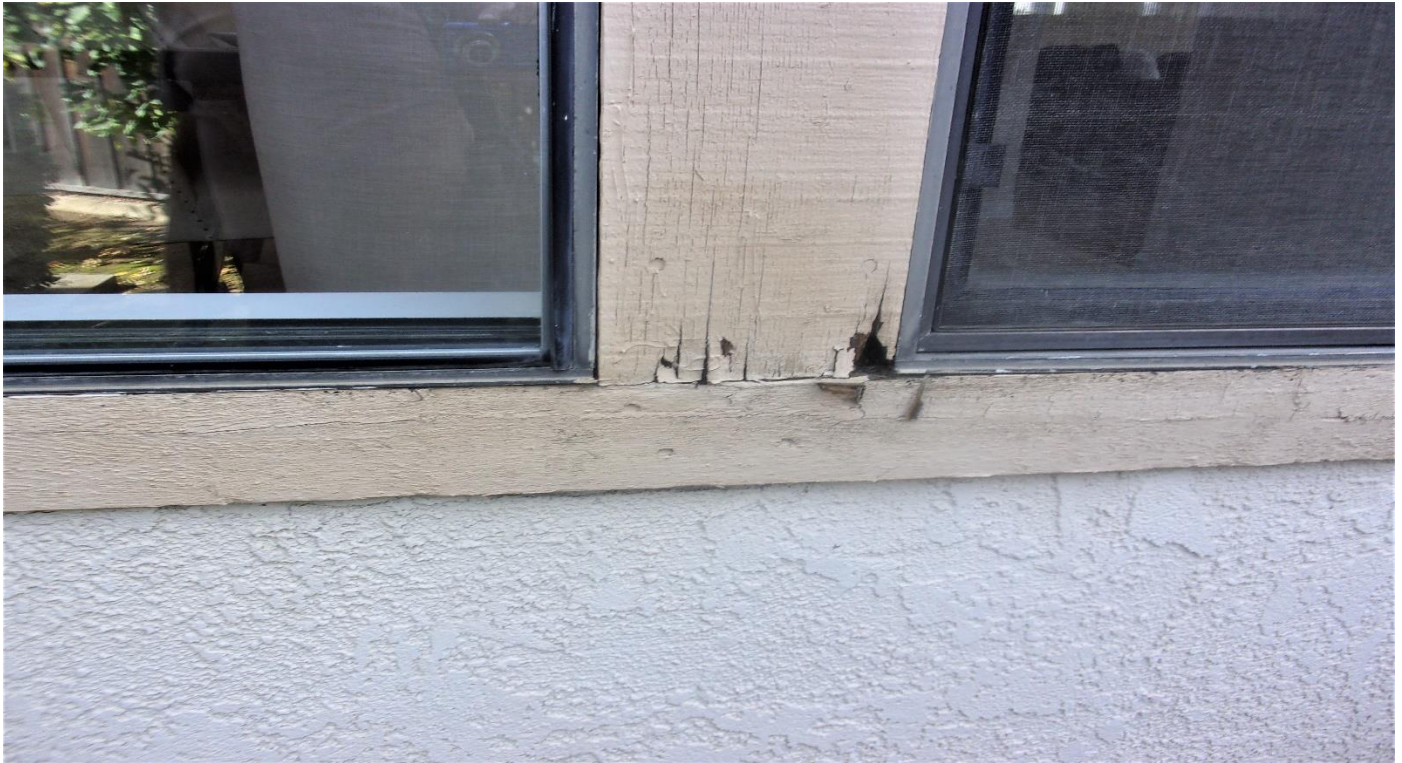
Moisture damaged wood window trim at east side of home.
