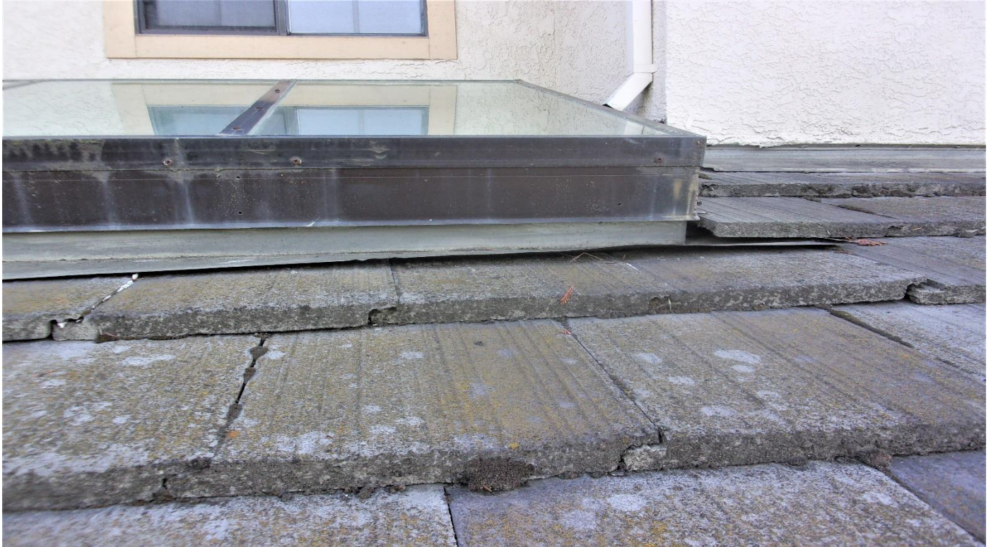
Loose flashing at roof surface.
