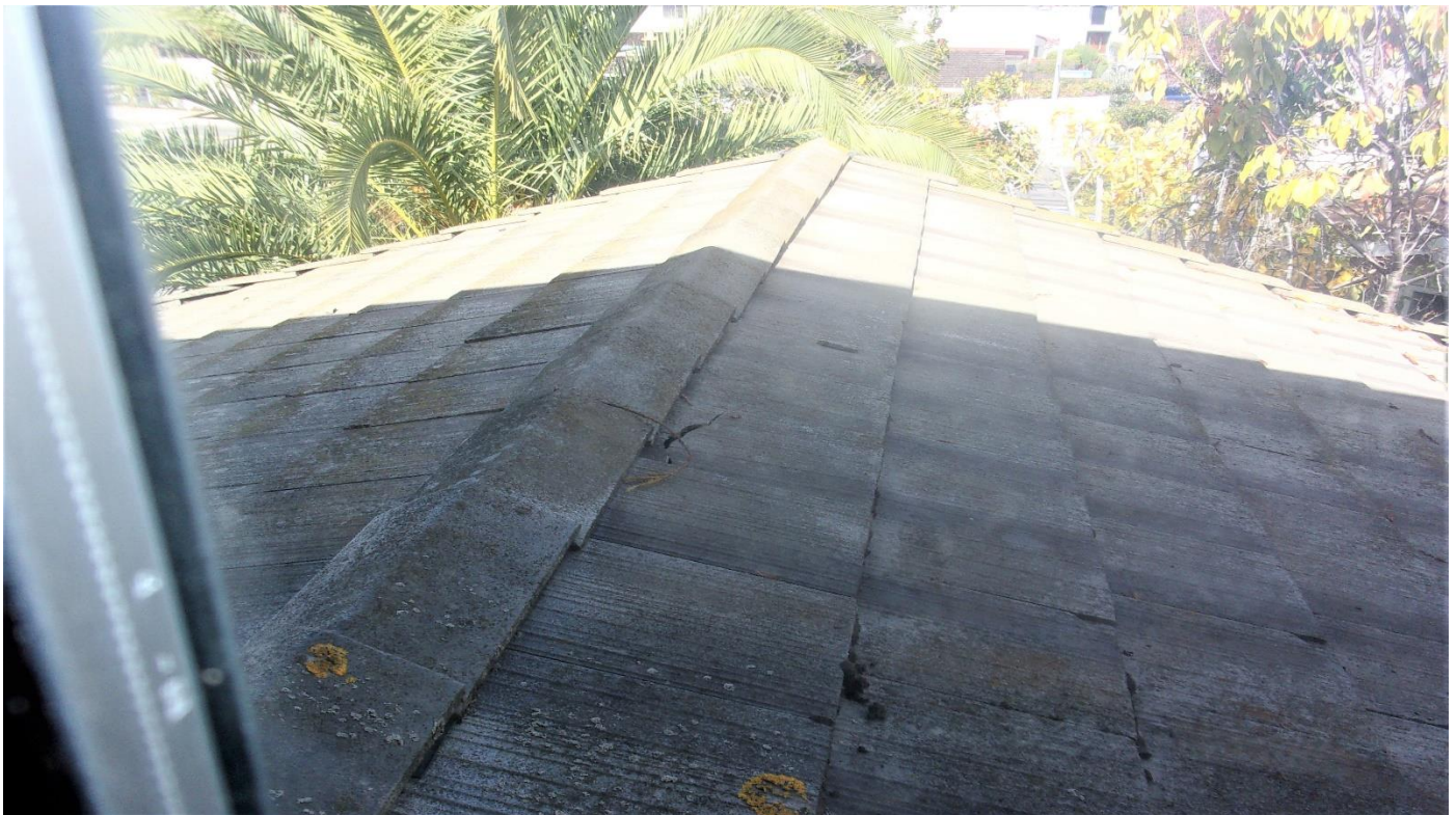
Cracked roofing tile visible at center of frame.
