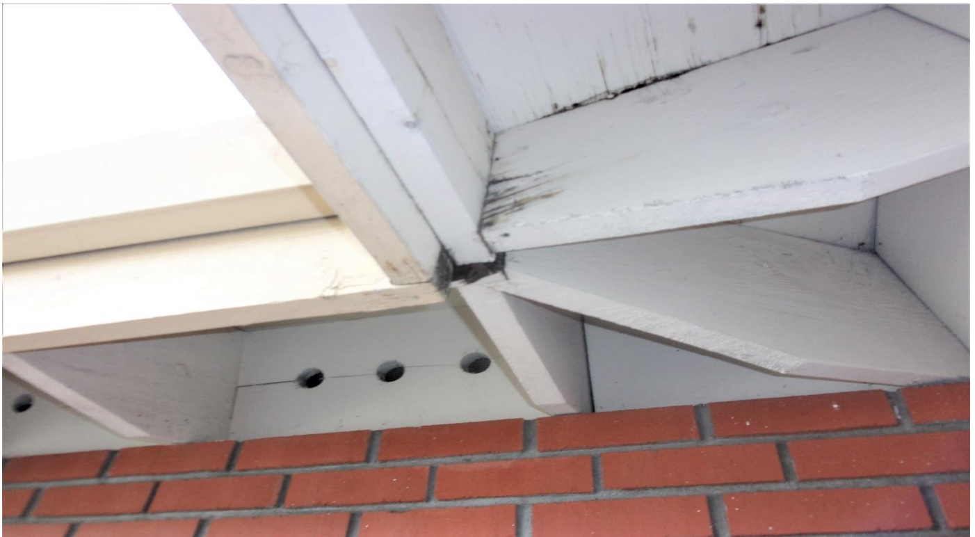
Moisture damaged wood at front lower level eaves.
