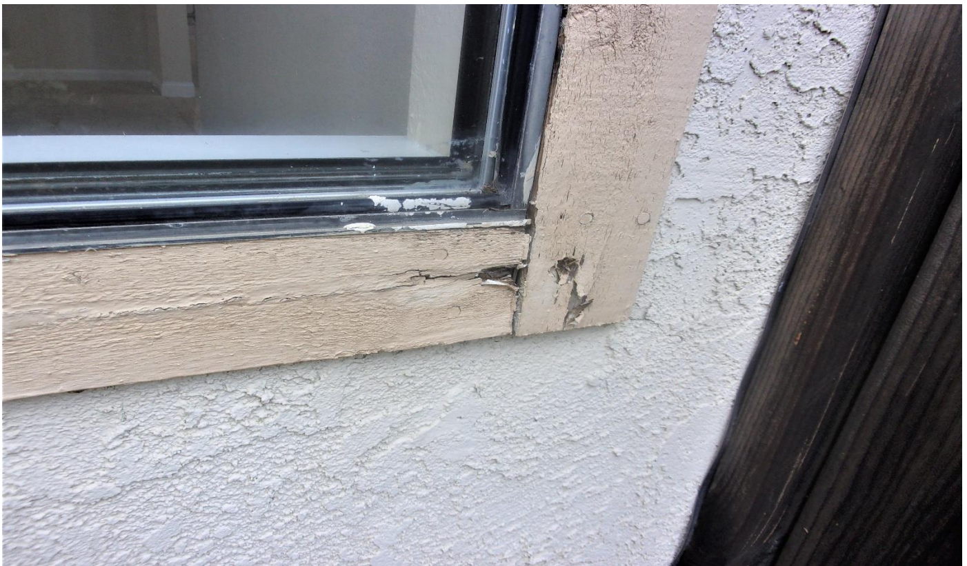
Moisture damaged wood at east side of home.
